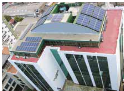
40KW solar net metering system at Millennium House complex at Navam Mawatha, Colombo 02
